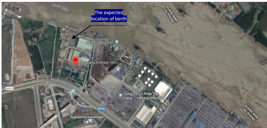
Figure 7: Location of the berth of Company Limited 189 in Cat Hai - Dinh Vu Economic Zone
