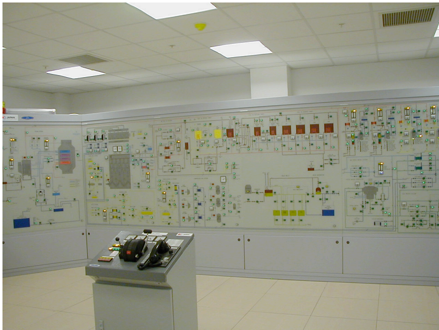
Fig.1 The former mimic panel
