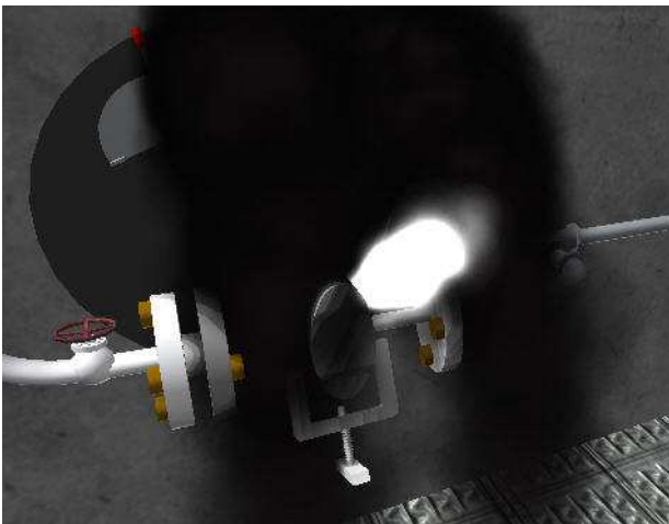
Figure 6 Steam and oil spray if the user neglects to turn off the flow of fuel and steam before loosening the burner clamp.
