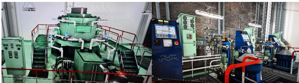
Figure 4. Steering gear and the purifiers in the marine engine room simulator (left to right).
